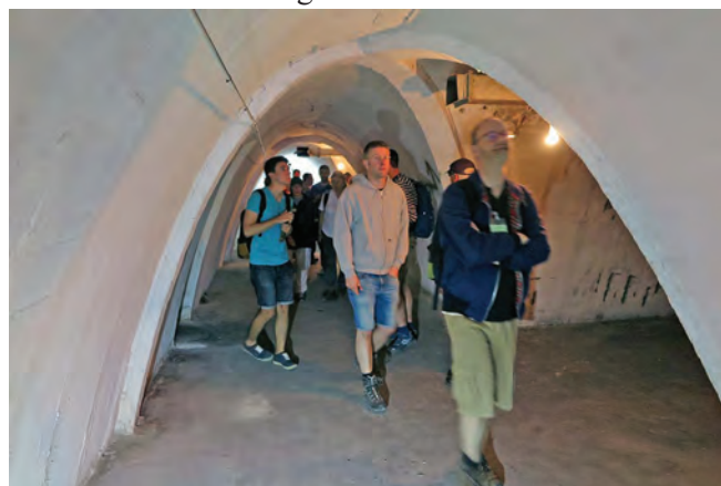
Crossover in the Tamariska Shelter shows the extra reinforcement at junctions
